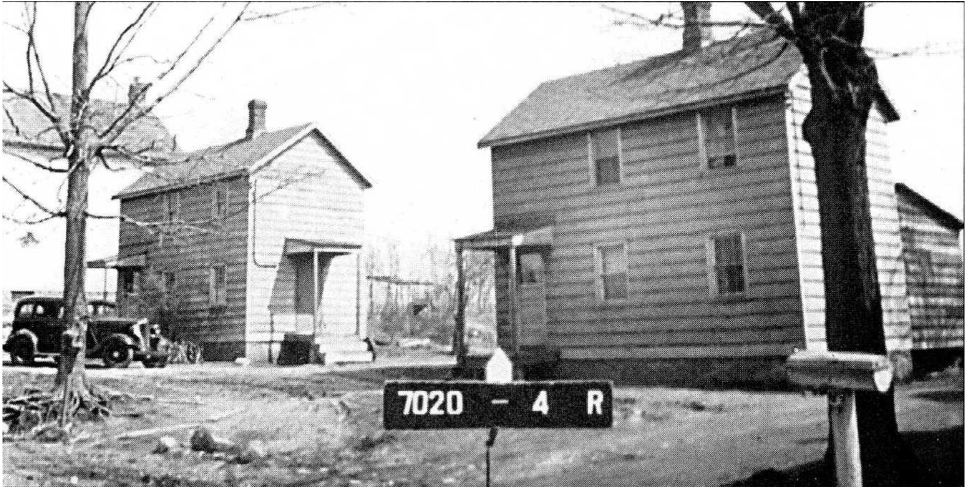
565 and 569 Bloomingdale Road Cottages Photo: New York City Department of Taxes (c. 1940), Municipal Archives
