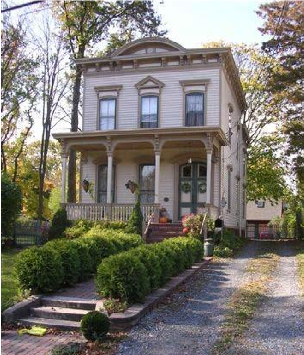
John H. and Elizabeth J. Elsworth House 90 Bayview Avenue Staten Island
